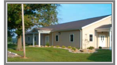
Southern Indiana Purdue Ag Center Agriculture Building
