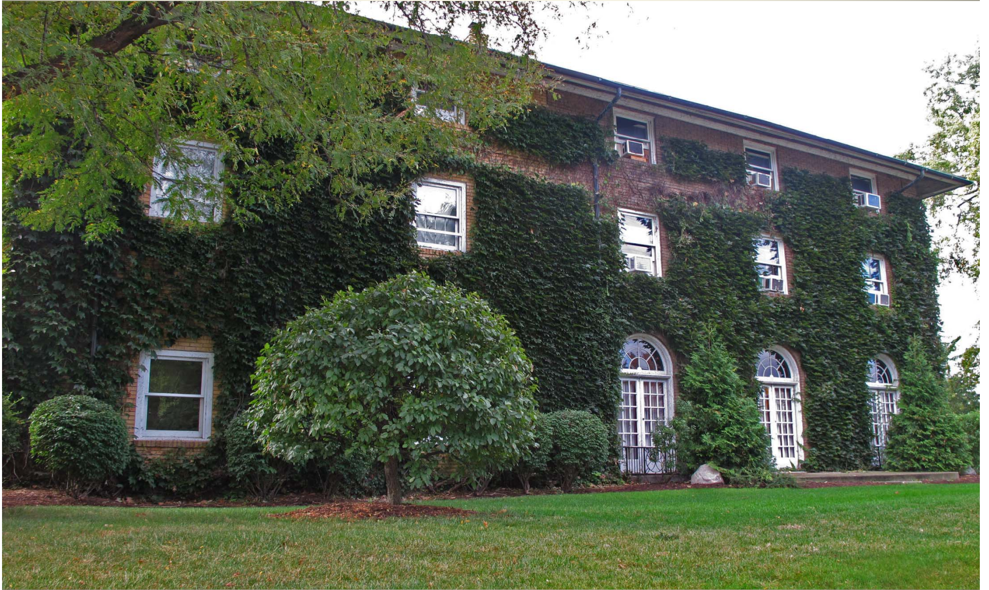
Ivy house at Stadium Ave.
